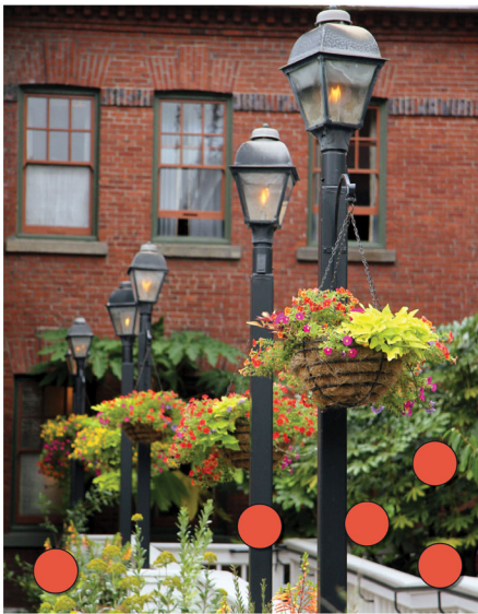
PEDESTRIAN STREET LIGHTING WITH PLANTERS
